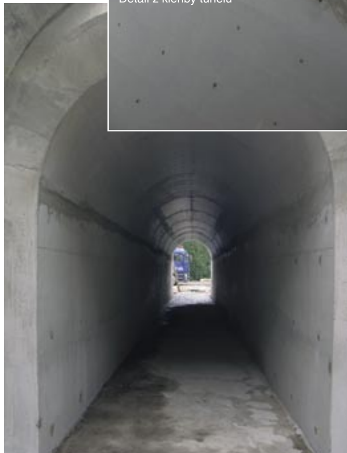
Detail z klenby tunelu
